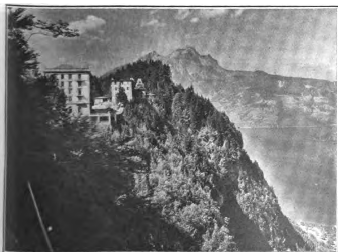
The Burgenstock, on the Lake of Lucerne, showing the Palace Hotel, which the Swiss Automobile Club visited
